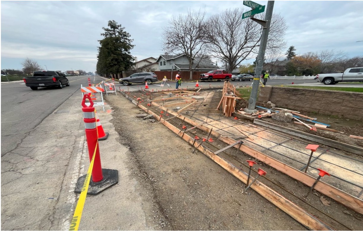
Construction at Ward and Mackilhaffy
