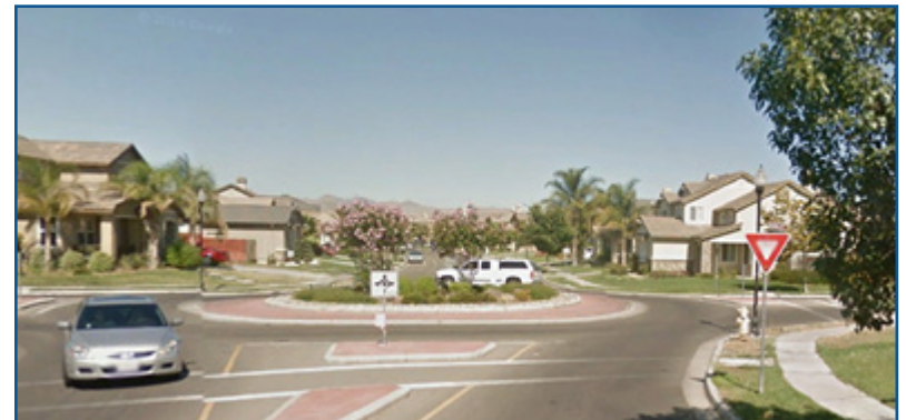
Bulb-outs with landscaping and decorative paving
