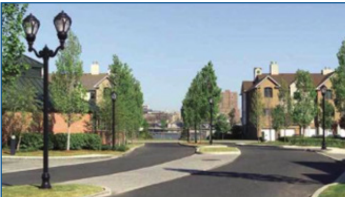
Double-headed decorative lighting along collector street
