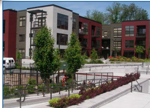
Apartments with varied rooflines and building articulation
