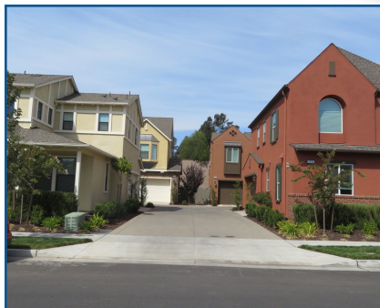
Auto court clusters with attractive landscaping and lighting
