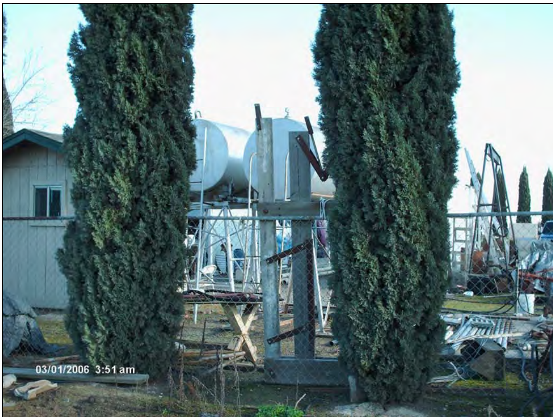
Figure 6-8. View Looking South of Two ASTs (APN 047-031-013)
