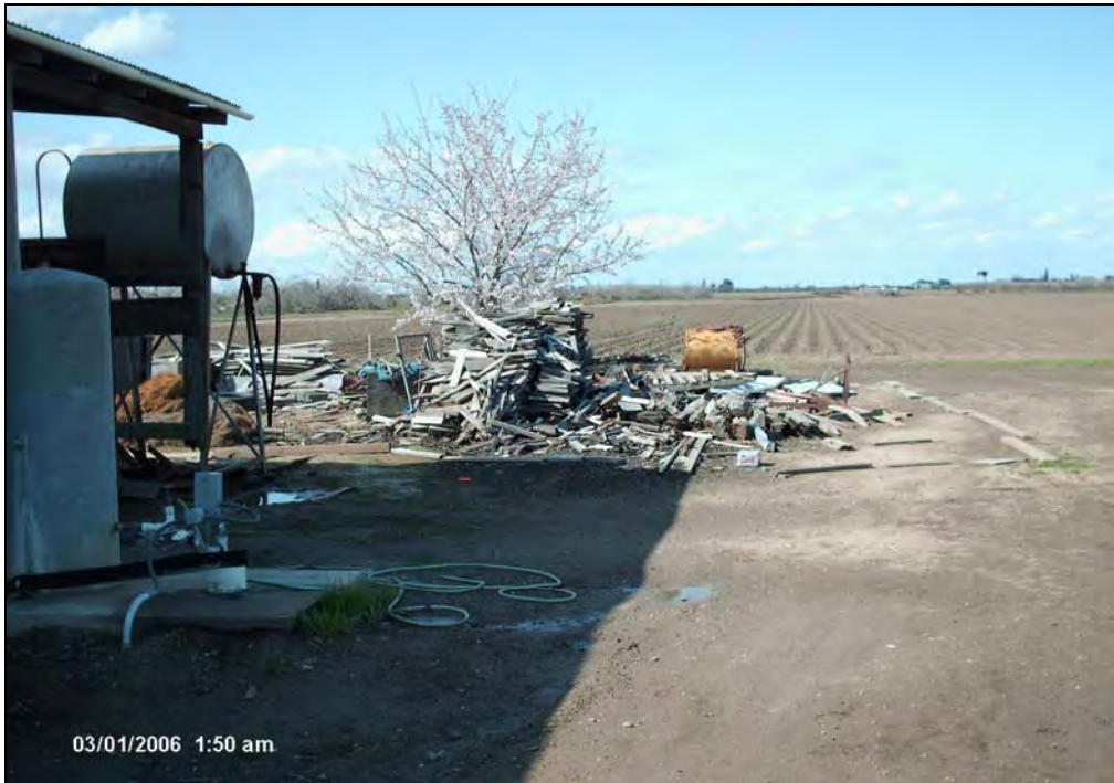
Figure 6-6. View Looking North at Same AST in Shop and One Beyond (APN 047-025-035)
