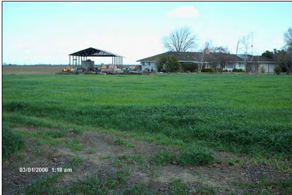
Figure 6-9. View Looking East of Filice's Property, with 3 ASTs Visible under Pole Barn (APN 047-025-014)
