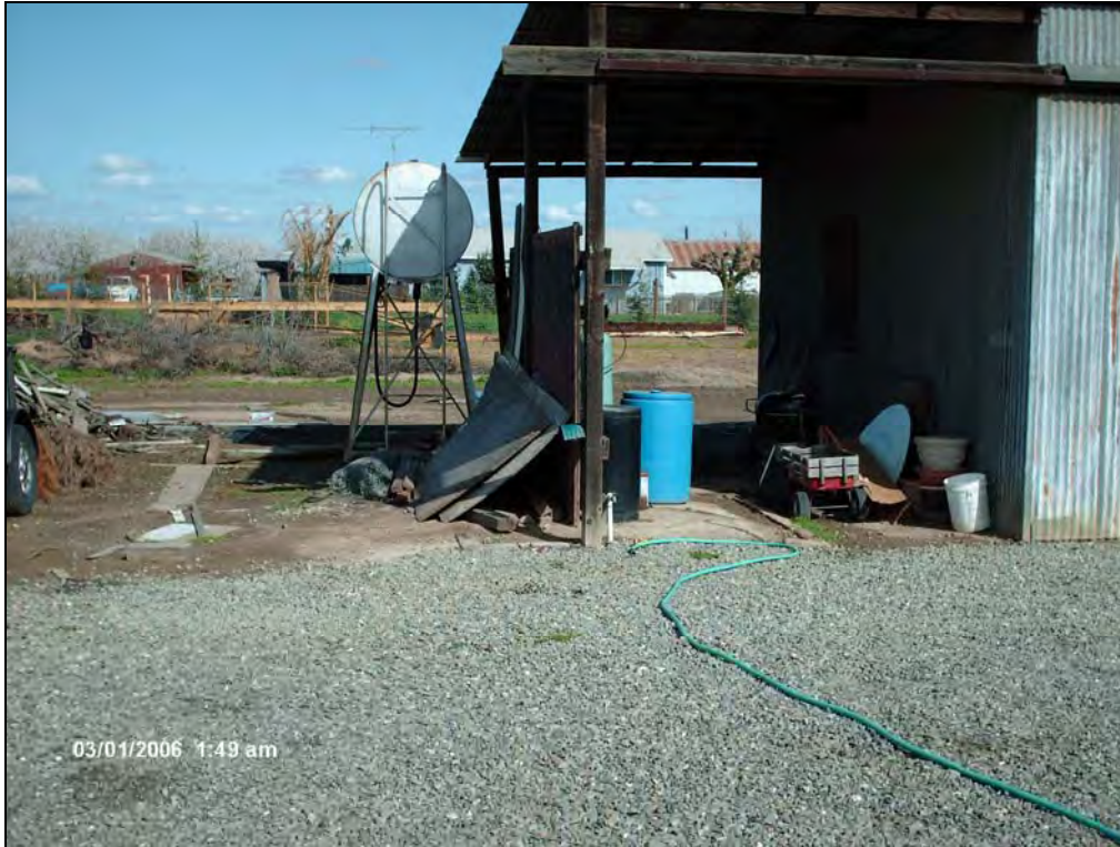
Figure 6-5. View Looking East of AST and Shop (APN 047-025-035)
