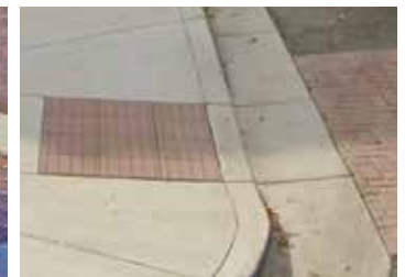
Example of ADA ramp improvements
