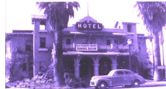
An example of the eclectic mix of architectural styles in the downtown, the Del Puerto Hotel was destroyed by fire in 1996.
