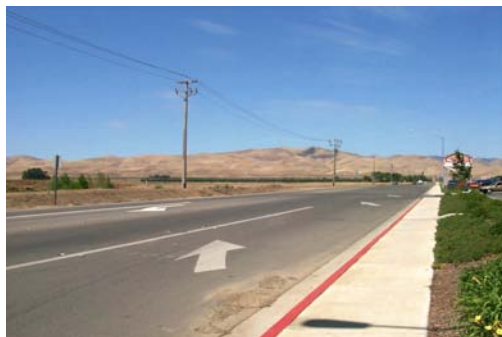
Sperry Avenue looking west in front of new commercial development.
