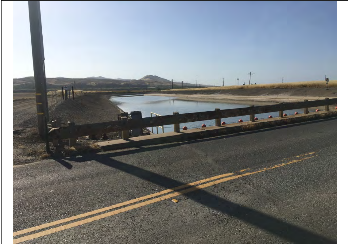
View of the Delta-Mendota Canal, facing northwest.
