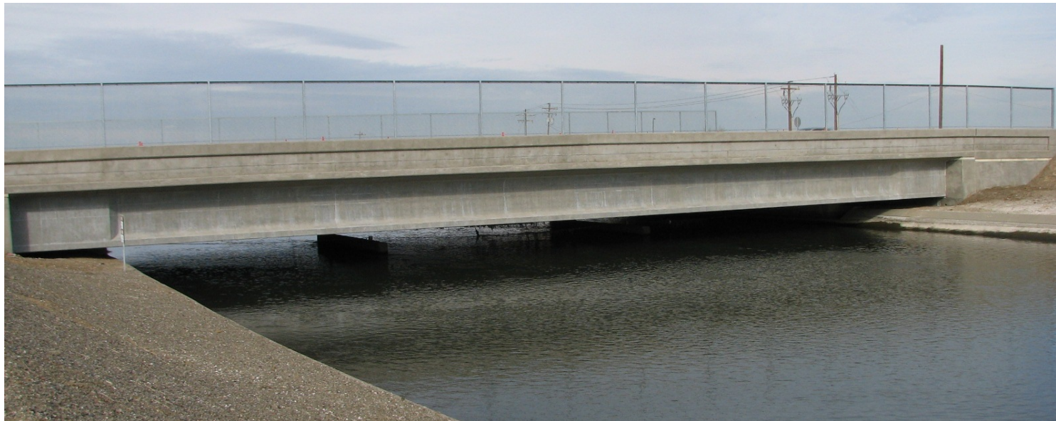
Sperry Road over Delta-Mendota Canal
