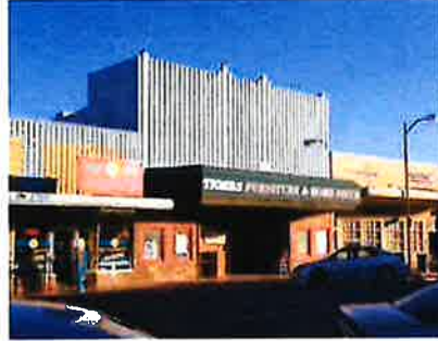
FURNITURE STORE IN OLD THEATER BUILDING
