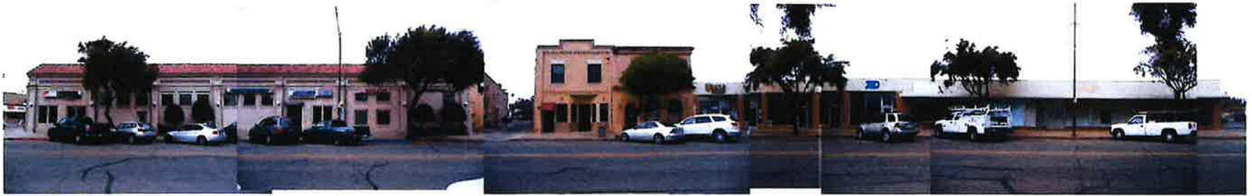
N. 3rd Street - west side.
