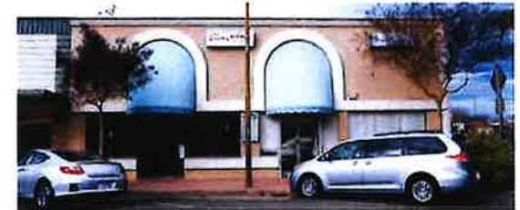
A historic building on S. Del Puerto that was covered with a stucco facade that does not reflect the historic architectural character.
