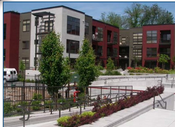
Apartments with varied rooflines and building articulation
